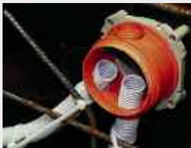
Flexible pipes installed into KBT body.
