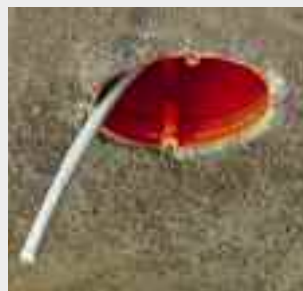
The KBT... box with terminated conductor ready for mounting the KBP... chandelier hook.
