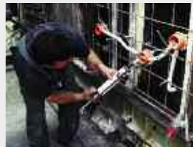
Sealing the penetrations (mastic).
